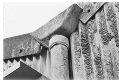
Asbestos cement down-pipe, hopper and sheeting
