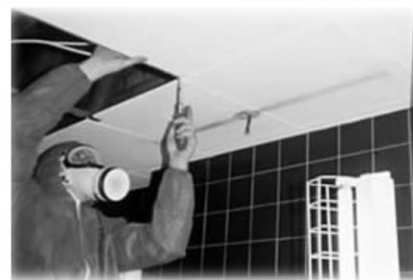
Unscrewing AIB ceiling boards
